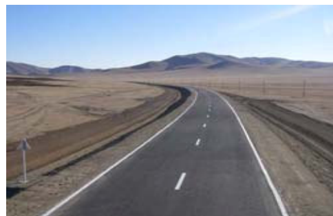
Picture 7. Part of road under construction
